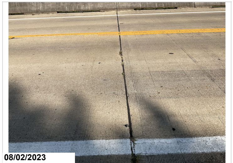
Joint material Bent 4 worn
