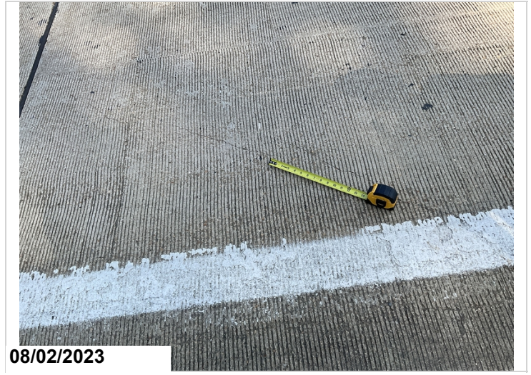
Deck cracks span 6 up to 0.020"
