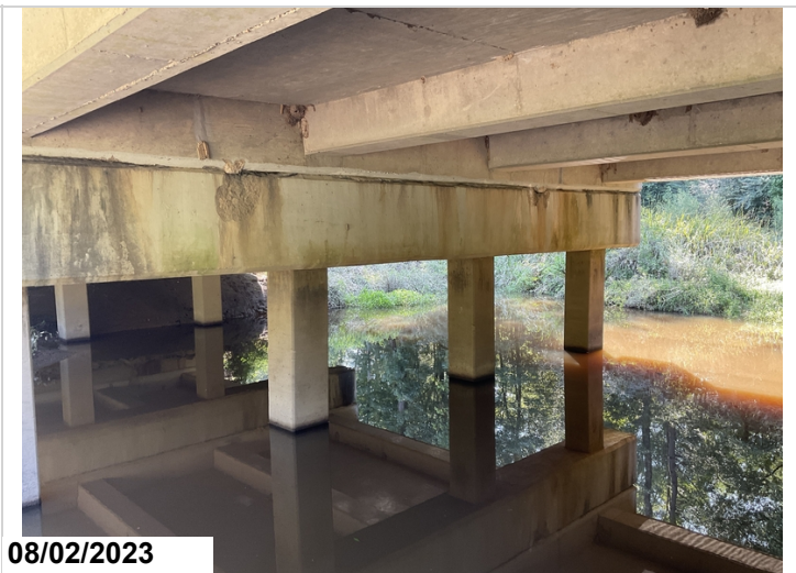
Bent 5 cap back spalls
